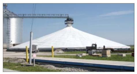
Closeup of the smaller of two LeMar center fill temporary storage piles. This one is 250 feet in diameter and holds about 1 million bushels. Newest Weigh Tronix truck scale is in the foreground.
