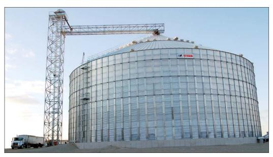
Above, new Chief Titan 1.1-million-bushel tank, with its own receiving pit and leg, installed in 2007 at United Cooperative's South Beaver Dam elevator in Wisconsin. At right, a view of the entire elevator. Photo above courtesy of United Cooperative; all other photos by Ed Zdrojewski.
