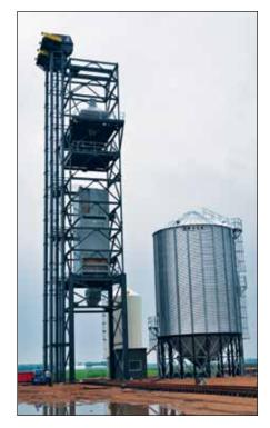
Intersystems screener and bulk weigh scale are housed in a separate Warrior support tower directly over the loop track and are fed from a below-ground Schlagel enclosed belt conveyor and jump leg.
