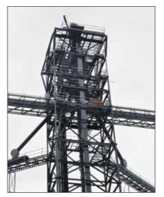
Receiving legs feed into a five-hole Schlagel electronic triple distributor.
