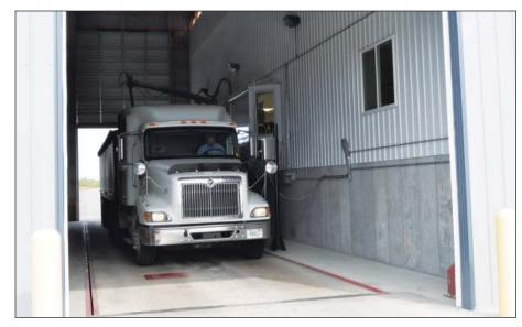
An incoming grain truck is weighed and probed in an enclosed scalehouse bay.
