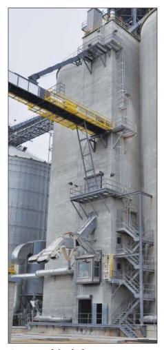
A portion of the slipform concrete structure houses a 80,000-bph Intersystems bulk weigh loadout scale that has loaded 110-car trains in less than six hours.
